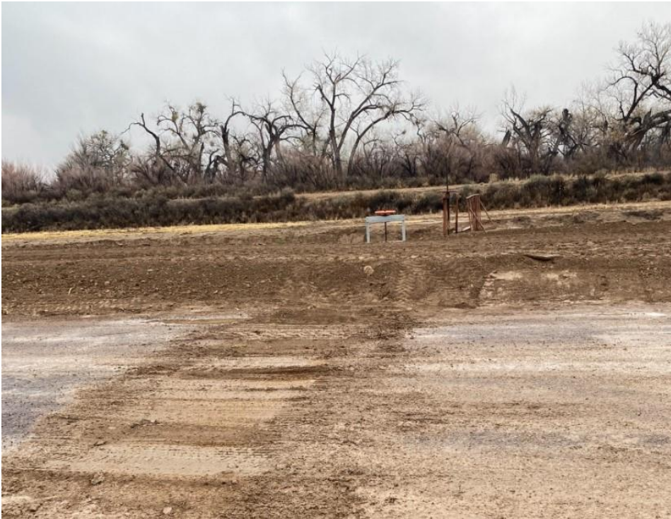
Newly replaced irrigation turnout.
