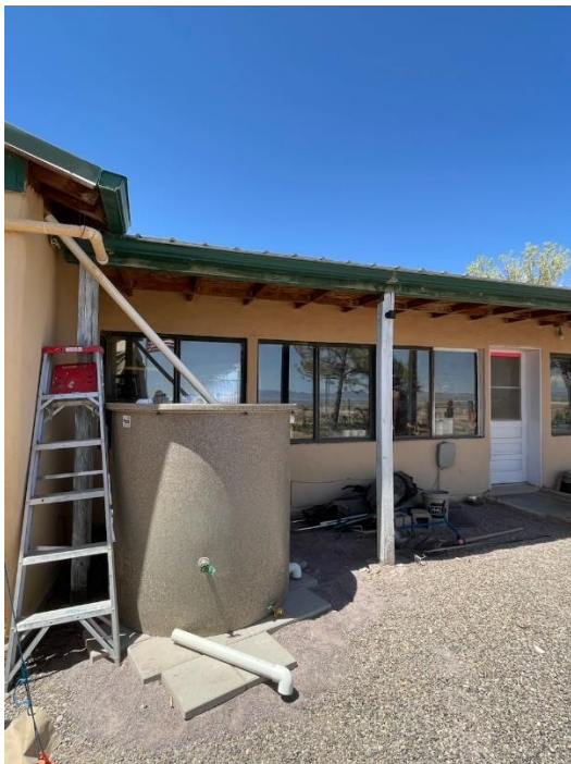
Rainwater harvesting barrel.
